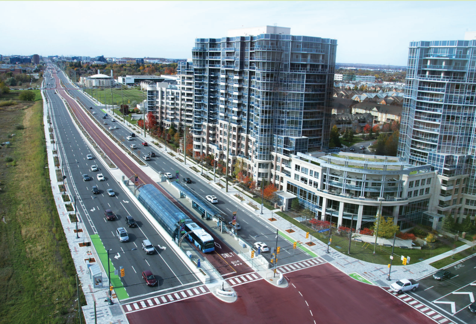
Red-tinted pavement along the Highway 7 East rapidway in Markham.
