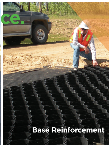
Subgrade Stabilization
