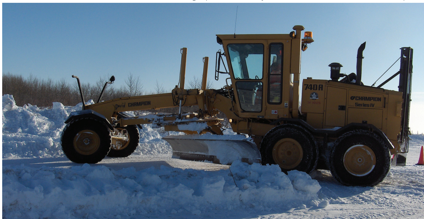
Snow removal on James Bay Winter Road
