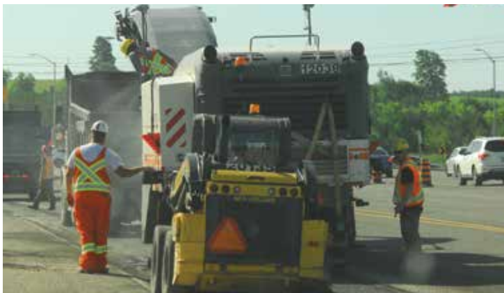
3D milling allows milling road crews to work with less material to complete the job.
