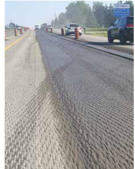
The cutting-edge 3D milling technology allows for variable milling depth on a road, resulting in perfect smoothness.
