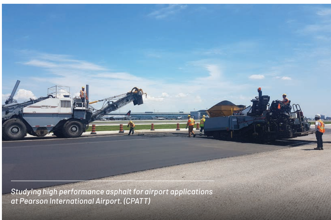
Testing the stability of asphalt mixes with recycled concrete aggregates. (CPATT)
