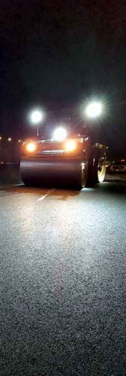
The P-404 surface course was 50 mm thick after compaction. (McAsphalt)
