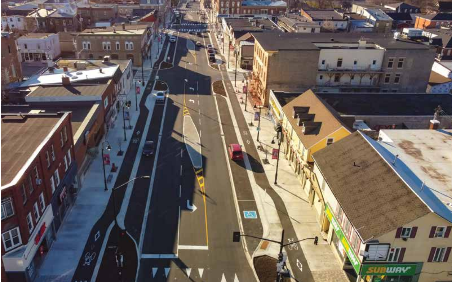
Beckwith Street, Smiths Falls. (Tomlinson)
