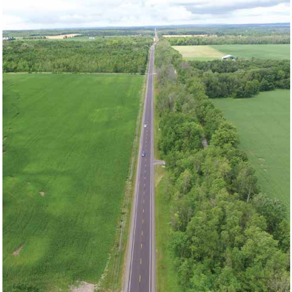
Simcoe County Road 6. (Coco Paving)
