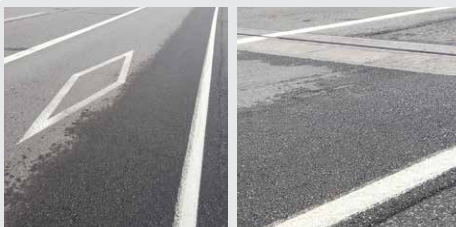
Figure 3. Ottawa bus lane shows no rutting after two summers even at bridge deck expansion joint.
