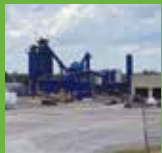
D. CRUPI & SONS LTD. Oshawa Asphalt Plant
