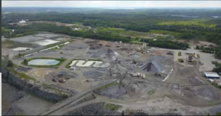
FOWLER CONSTRUCTION COMPANY LTD. Rosewarne Asphalt Plant
