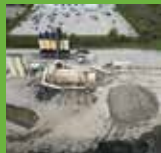
BRANTCO ASPHALT AND MATERIALS LTD. Cambridge Asphalt Plant
