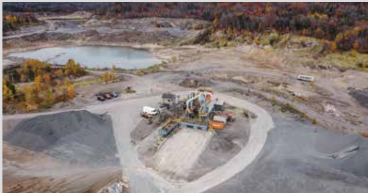
ELLWOOD ROBINSON INC. Ellwood Robinson Asphalt Plant
