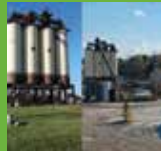
GREEN INFRASTRUCTURE PARTNERS (GIP) INC. Kitchener Asphalt Plant
