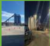
D. CRUPI & SONS LTD. Passmore Asphalt Plant
