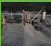
GREEN INFRASTRUCTURE PARTNERS (GIP) INC. Boyce Asphalt Plant
