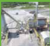
GREEN INFRASTRUCTURE PARTNERS (GIP) INC. Kemptville Asphalt Plant
