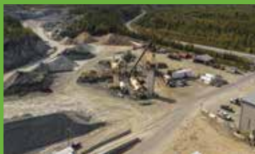
GREEN INFRASTRUCTURE PARTNERS (GIP) INC. - GIP Interpaving Garson Asphalt Plant – Sudbury
