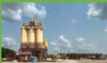
THE MILLER GROUP Richmond Hill Asphalt Plant #2
