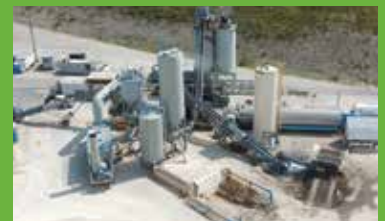
HAROLD SUTHERLAND CONSTRUCTION LTD. Downs Pit Asphalt Plant
