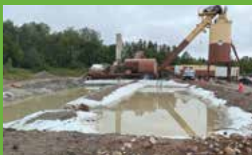
THE MILLER GROUP Foleyet Asphalt Plant #19
