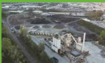
STEED AND EVANS LTD. Cambridge Asphalt Supply Plant
