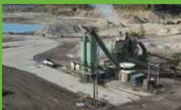
STEED AND EVANS LTD. Heidelberg Asphalt Plant
