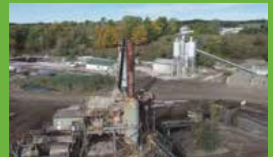
GREEN INFRASTRUCTURE PARTNERS (GIP) INC. Guelph Asphalt Plant
