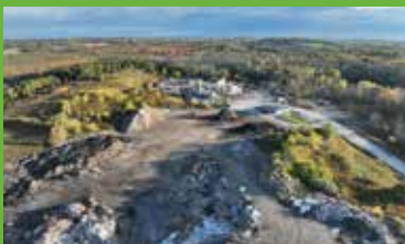
GREEN INFRASTRUCTURE PARTNERS (GIP) INC. Peterborough Asphalt Plant
