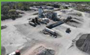
GREEN INFRASTRUCTURE PARTNERS (GIP) INC. Westbrook Asphalt Plant
