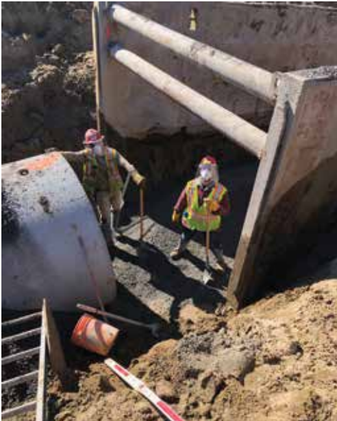
Construction workers attired in PPE
