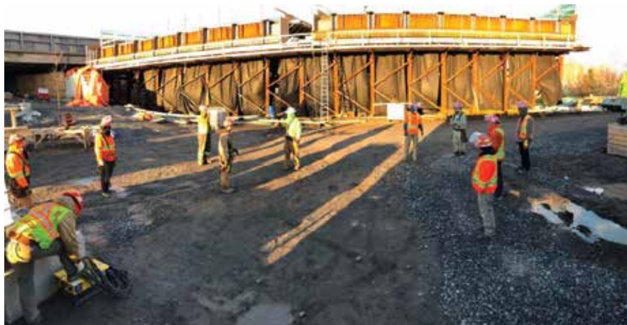
R.W. Tomlinson workers practising social distancing at a job site
